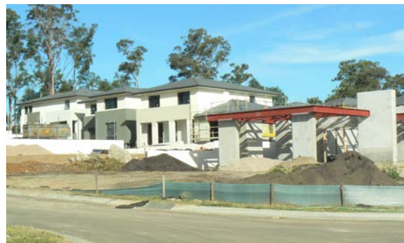
Gilroy College Target site under construction
