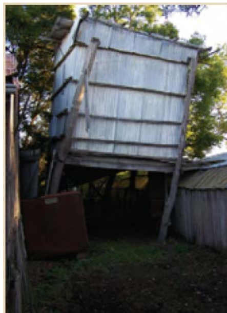
Funding provided to complete conservation works at St Elmo Dural
