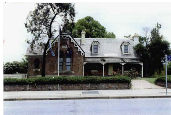
Former Castle Hill Public School Source: Baulkham Hills Heritage Study 1993-1994
