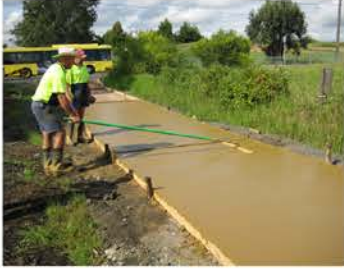
Construction of new track
