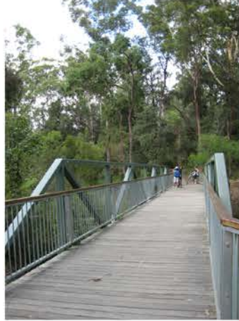
Bridge over Smalls Creek
