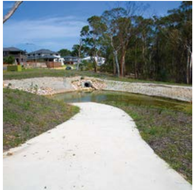
Bladensburg Road Reserve, North Kellyville – detention basin
