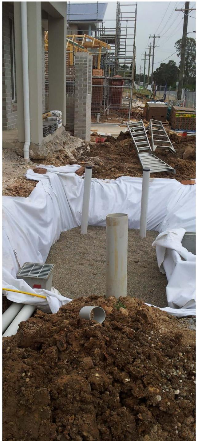
29. The area underneath the "surcharge pit" must be filled using clean, fine gravel similar to that used in the "drainage layer" (see below).
